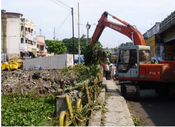
Pre-Monsoon works at Jaffarkhanpet bridge in Adyar river
