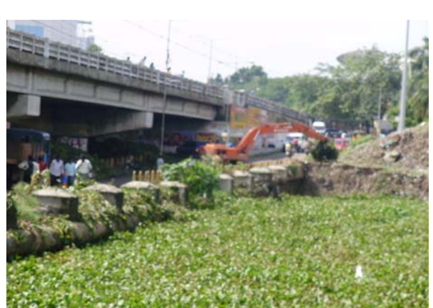
Pre-Monsoon works at Jaffarkhanpet bridge in Adyar river
