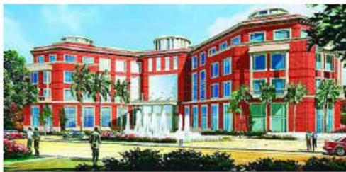
ITC GREEN CENTRE, GURGAON - PLATINUM LEED RATED
